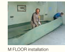
M FLOOR installation
